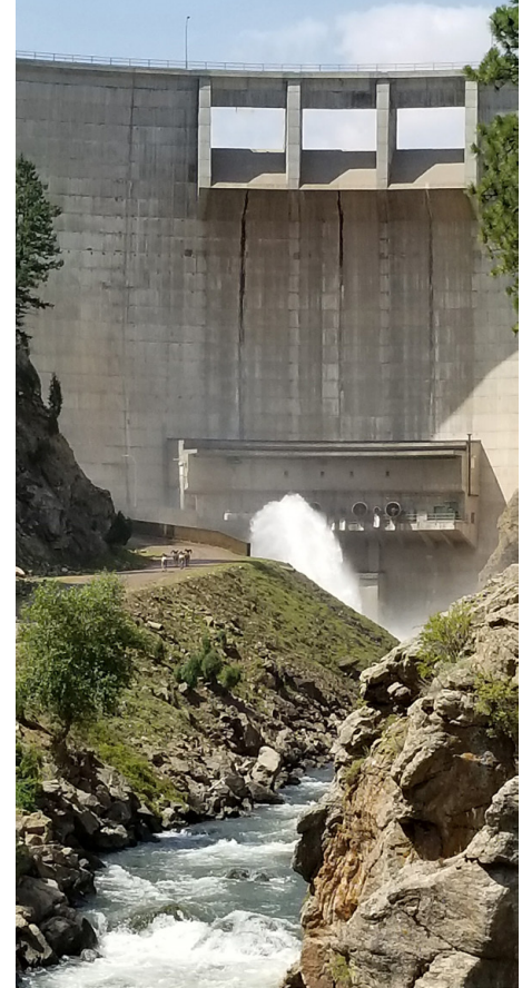
Denver Water’s Strontia Springs Dam on the South Platte River in Waterton Canyon.
